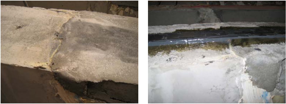
Figure 6-30. Left: Interface between original concrete and repair mortar. Right: CFRP plate bonded to the repaired beam.
