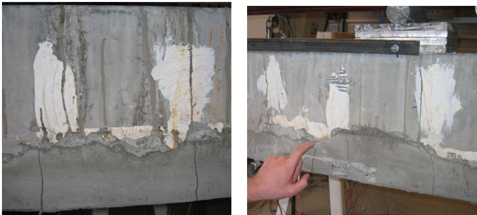
Figure 6-26. Large cracks formed in the repair mortar during failure test.
