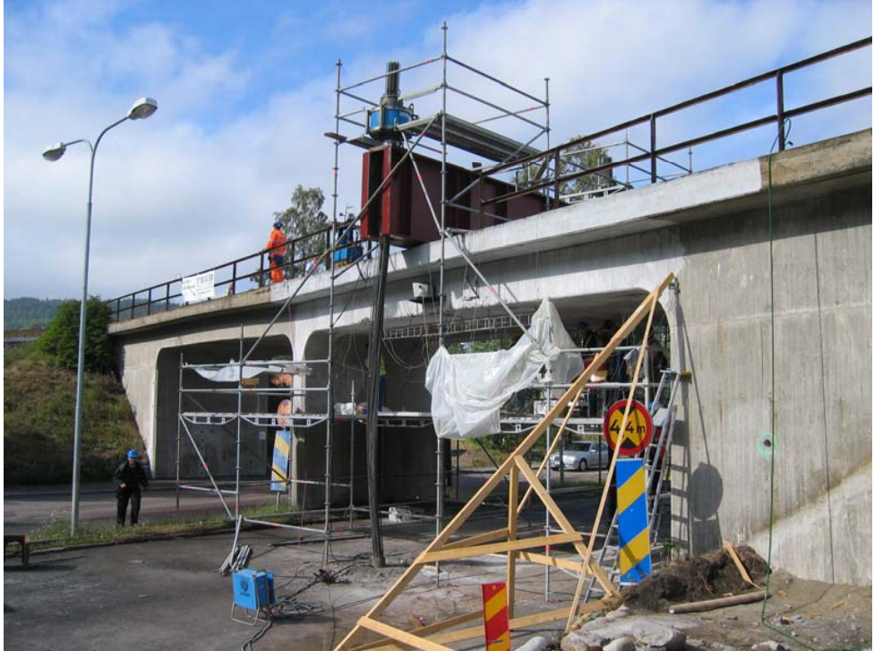
Figure 3-22. Ö-vik bridge in Sweden during failure test in the summer of 2006.
