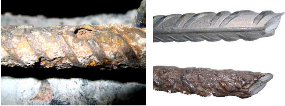
Figure 6-2. Left: Both evenly distributed corrosion as well as pitting corrosion was observed on corroded steel reinforcement bars. Right: Failure surface for corroded and undamaged steel reinforcing bars after material test.
