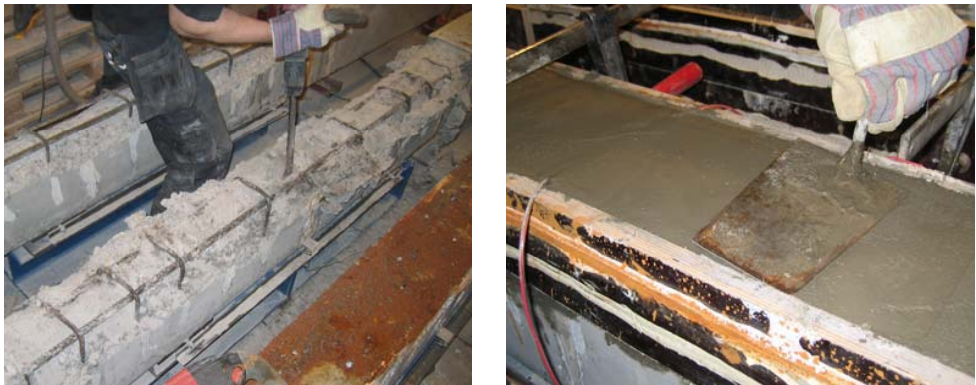
Figure 5-6. Left: Cover concrete was removed using jack hammer. Right: The cavity was refilled with repair mortar.
