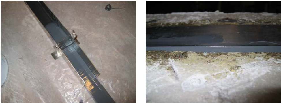
Figure 5-7. Left: Adhesive tool to apply the right amount of adhesive to the plates. Right: Concrete surface, adhesive layer and CFRP plate.
