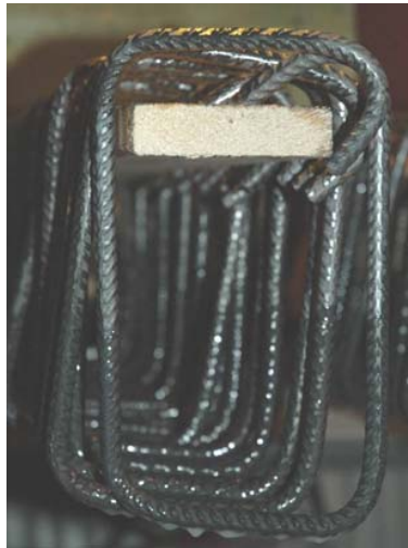
Figure 5-4. Stirrups were protected against corrosion with a coating of epoxy adhesive. Here they are seen when left to harden.
