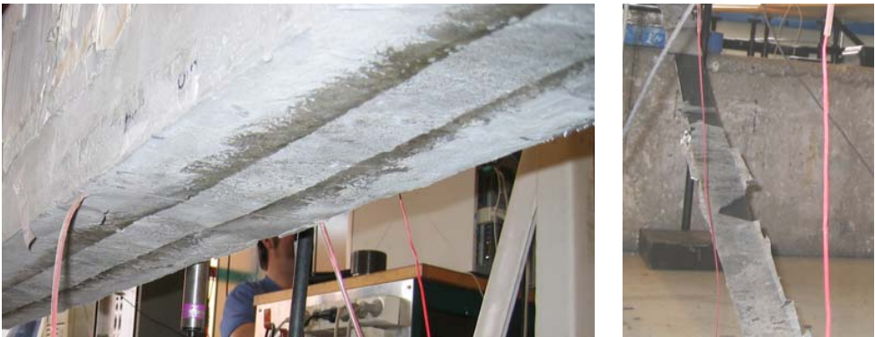
Figure 6-31. Left: The failure occurred in the interface between adhesive and concrete. Right: Only epoxy and primer was left on the CFRP plate after debonding.
