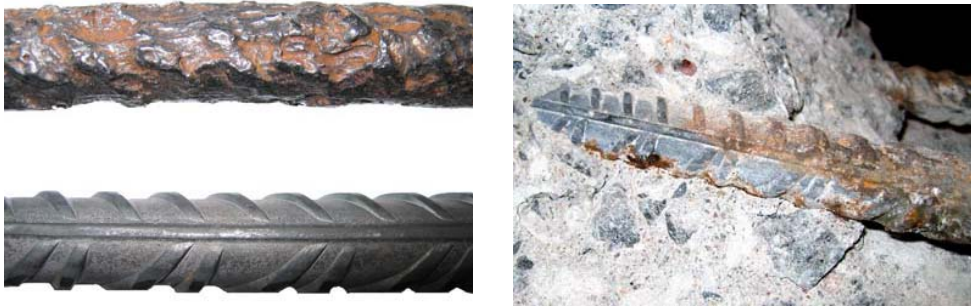
Figure 6-3. Left: Corroded and undamaged steel reinforcement. Right: The interface between the corroded and the undamaged steel section.
